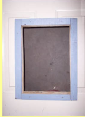
Installed door trim kit.
