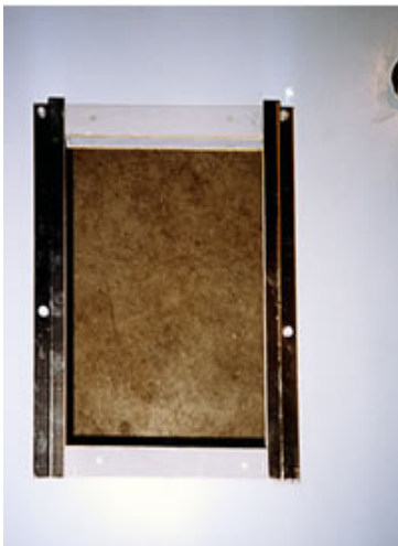
Install channel on inside of building Photo 1
